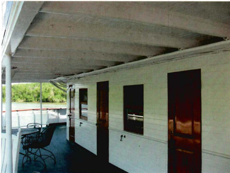
Condition of Wood Topsides – Typical - 5/2008
