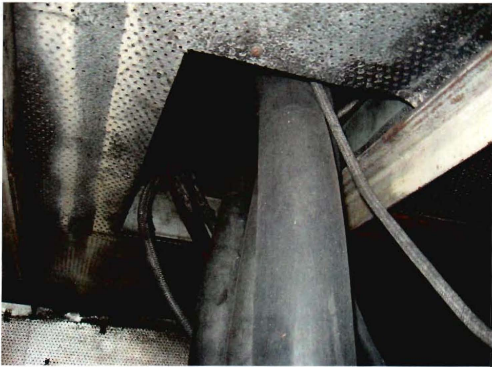
Steamer DELTA QUEEN CO2 Protected Generator Enclosures not Fume-tight -- 5/2008
