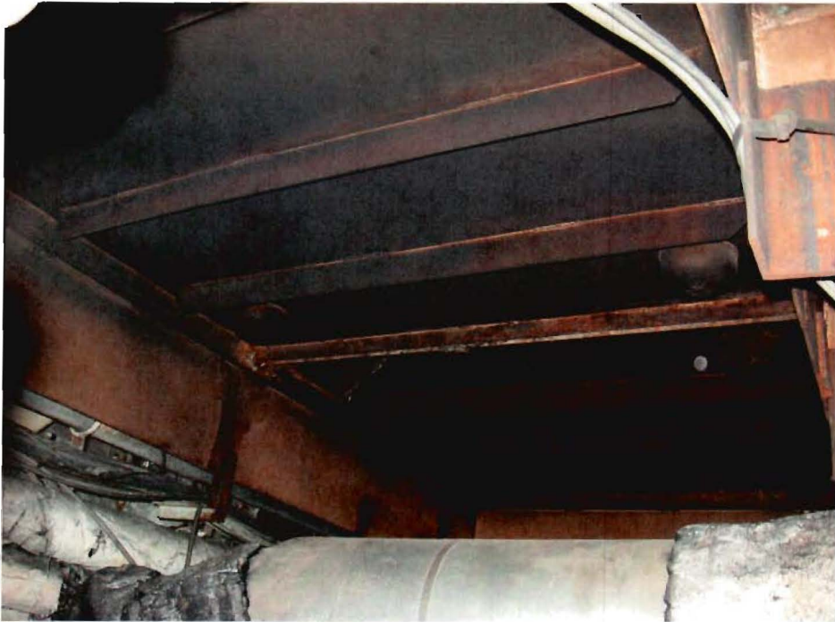
Below - Wood Underdeck over Starboard Generator Box with insulation
