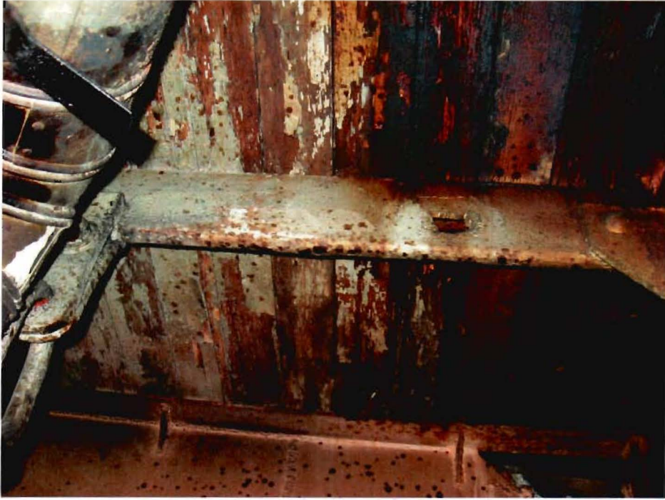
Above - Wood Underdeck over Port Generator Box without insulation
