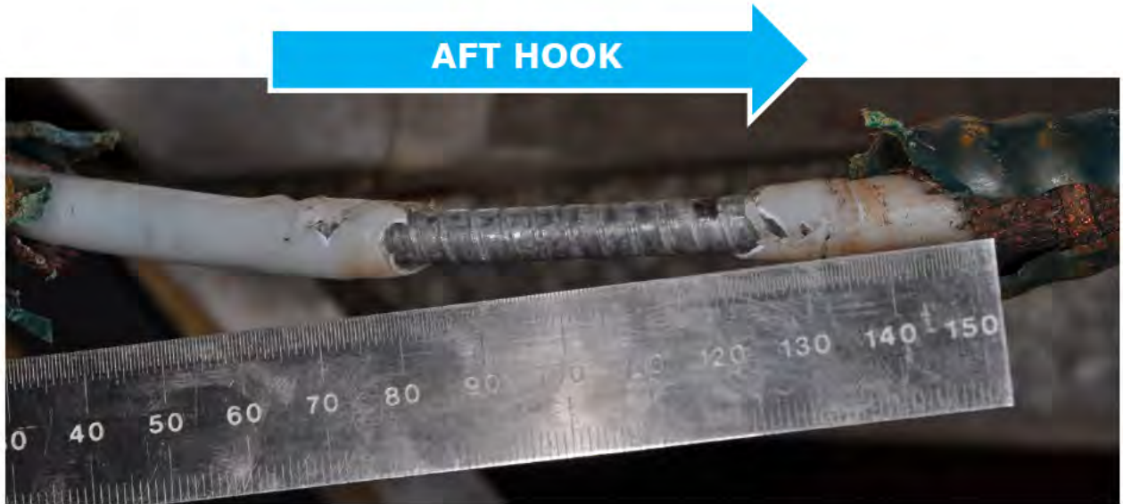
Figure 19. Photograph of the Subject Aft Cable showing a failure of the outer layers exposing the inner member. The direction of the Subject Aft Hook is noted with the blue arrow. Ruler is in mm.
