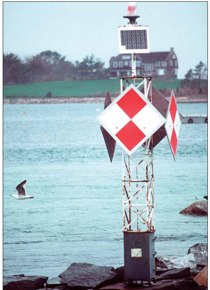
A solar-powered ATON. U.S. Coast Guard photo by Petty Officer Ron Mench.
