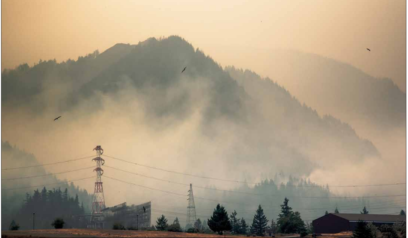
Heavy smoke from the Eagle Creek Fire hangs over the Bonneville Lock and Dam in September 2017. Mission-essential personnel remained at the dam to maintain safe operations and monitor the critical infrastructure. U.S. Army Corps of Engineers photo
