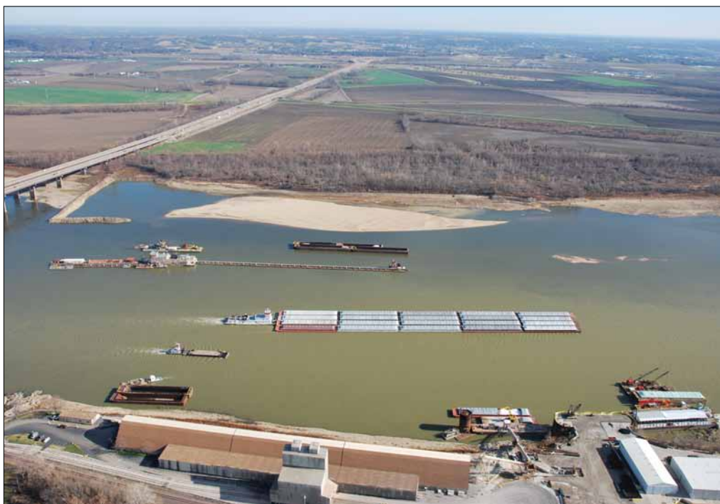
The U.S. Army Corps Dredge Potter works on the Mississippi just south of the Jefferson Barracks Bridge near St. Louis to ensure the channel is properly cleared and dredged in December 2012. Low water is also uncovering a sand bar near the southbound tow. Coast Guard photo
