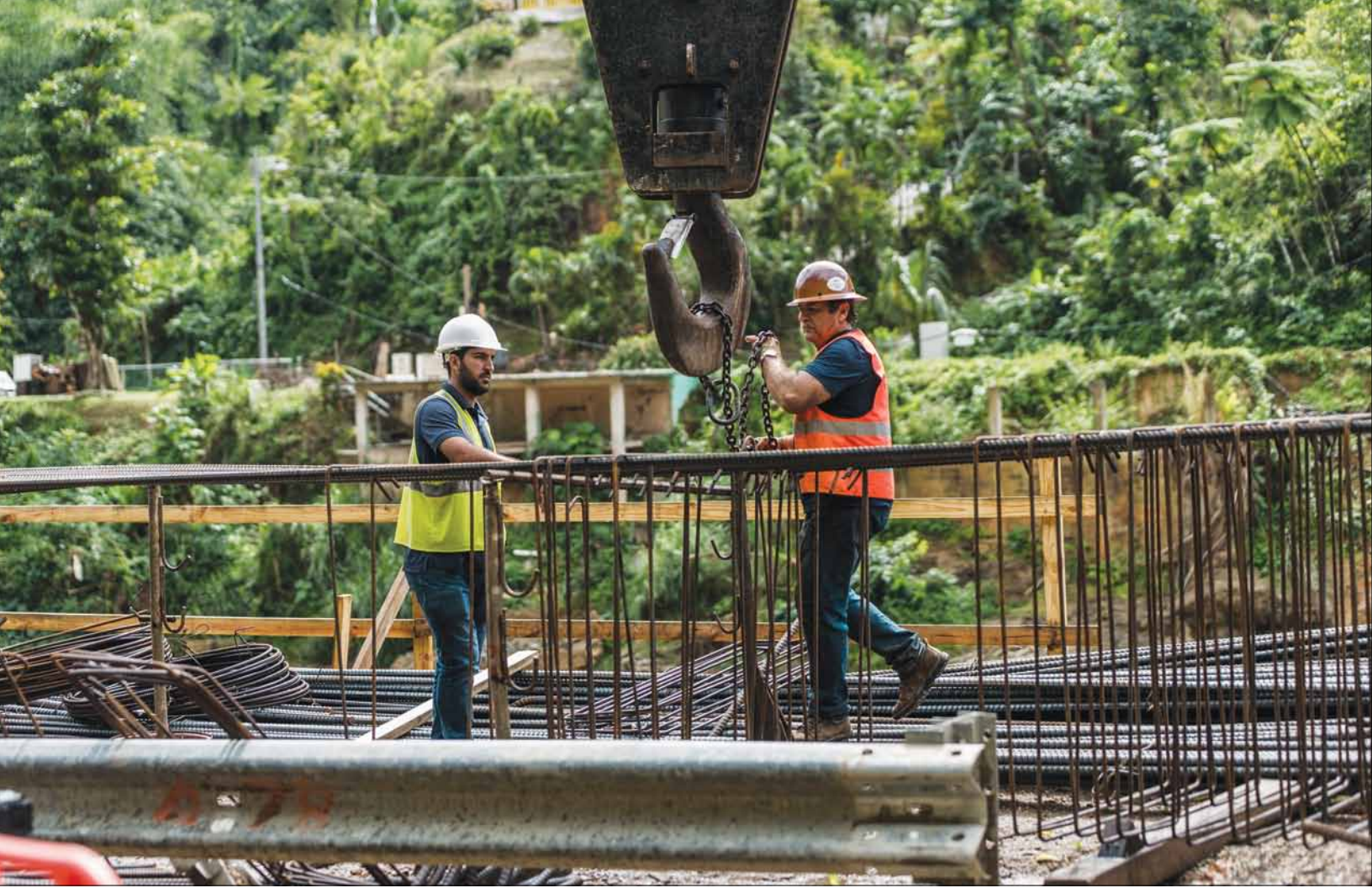
Workers tie rebar to set the foundation of the Río Abajo Bridge in Utuado, Puerto Rico, on January 27, 2018. The bridge collapsed due to debris from Hurricane Maria. FEMA photo
