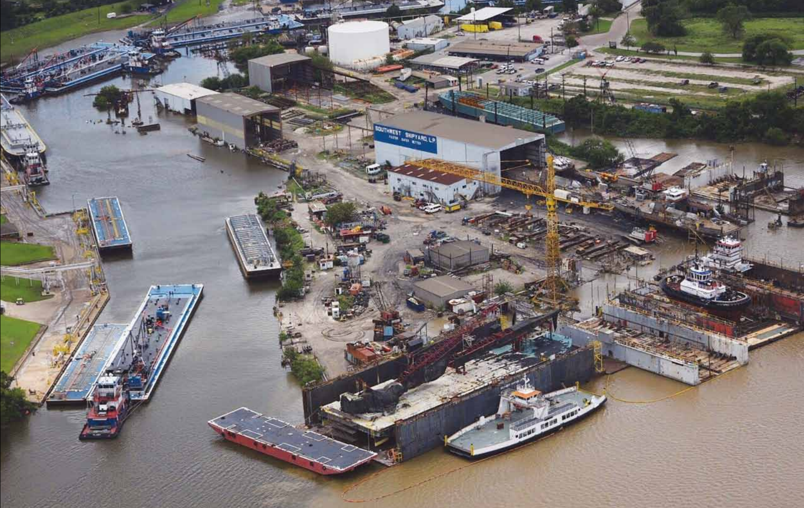
Coast Guard aircrews conduct flyovers to assess the ports of Houston, Texas City, Freeport, and Galveston, Texas in August 2017. These port assessments are conducted in order to identify any damaged Coast Guard-regulated port facility, potential oil spills, or chemical release as well as any navigational obstructions along the ports. Coast Guard photo by Petty Officer 1st Class Patrick Kelley
