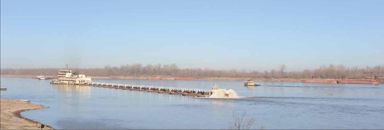
The Dredge Potter , one of the U.S. Army Corps of Engineers' dustpan dredges, removes sediment from the mainstem of the Mississippi River channel to keep commercial navigation flowing during extreme low-water conditions between St. Louis and Cairo, Illinois, in January 2013. Army Corps of Engineers photo
