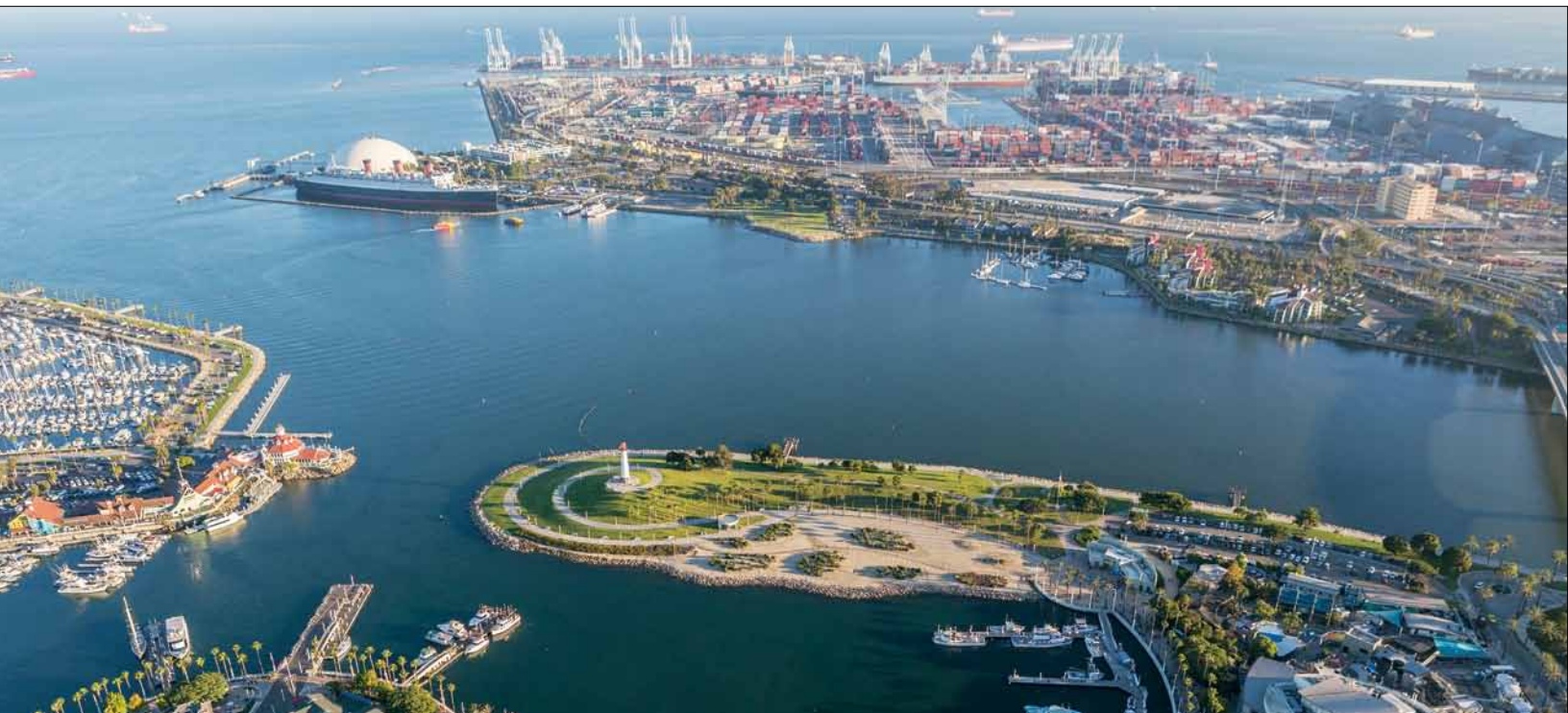
The busiest container port in the United States, the Port of Los Angeles, adjoins the separate Port of Long Beach. Together, these two port complexes cover nearly 4,300 acres of land and water along 43 miles of waterfront. Trekandshoot/Shutterstock.com
