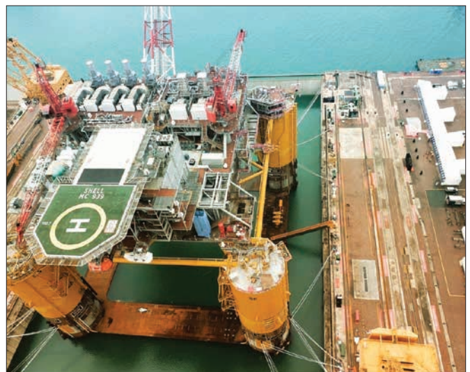
The Vito FPU is shown in Singapore in 2021 before the semisubmersible was delivered to Shell in December of that year. The FPU, the company's first deep-water platform in the Gulf of Mexico to employ a simplified, cost-efficient host design, went into production in Spring 2023 with an estimated peak production of 100,000 barrels of oil per day. Coast Guard photo by Mike Smith
