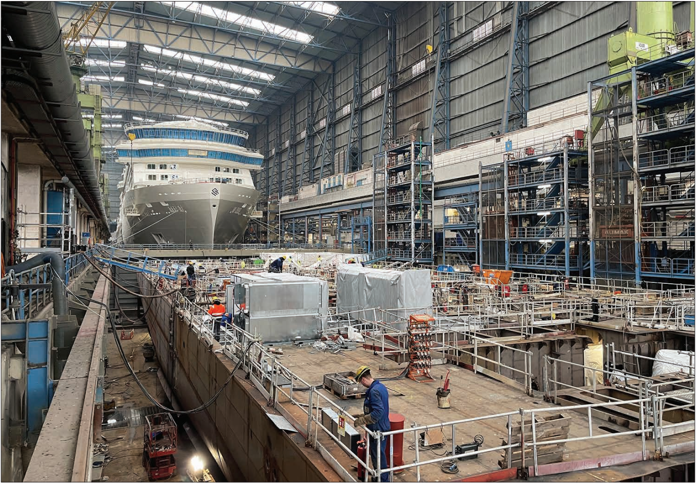
Meyer Werft's enclosed dry dock bay in Papenburg, Germany, allows for year-round construction. It is one of the largest facilities of its kind in the world and shields ships from rainy weather in Northern Europe. Coast Guard photo by LT Devin Greenwell
