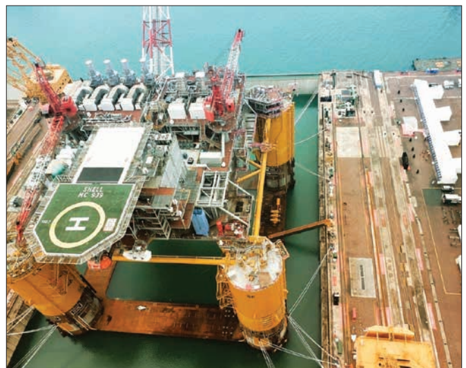
The Vito FPSO is shown in Singapore in 2021 before the semisubmersible was delivered to Shell in December of that year. The FPSO, the company's first deep-water platform in the Gulf of Mexico to employ a simplified, cost-efficient host design, went into production in Spring 2023 with an estimated peak production of 100,000 barrels of oil per day. Coast Guard photo by Mike Smith
